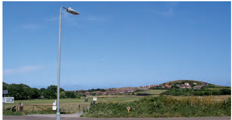
New low energy street lighting in Beeston Regis
